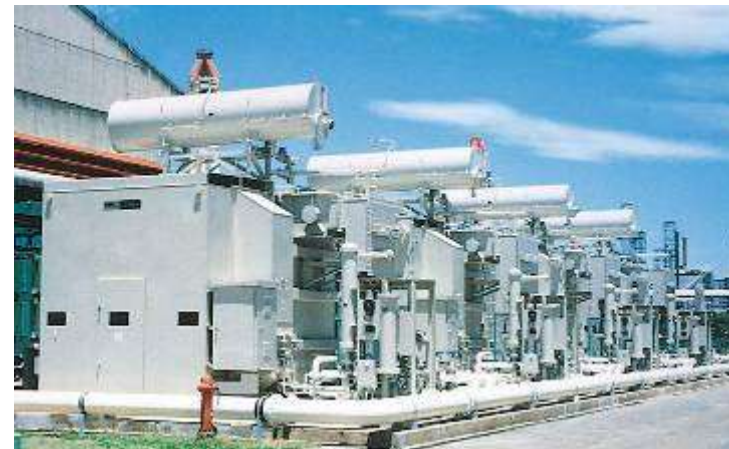
High-capacity rectification equipment
