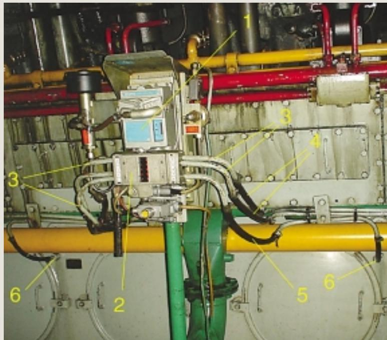
*Figure 7: Incorrect installation of an oil mist detector VISATRON® VN215 with individual suction pipe connected to each compartment for localization of damage*
