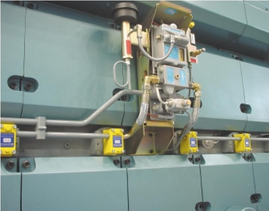
Figure 5: Classic oil mist detector provided with siphon block suction system for each crankcase compartment
