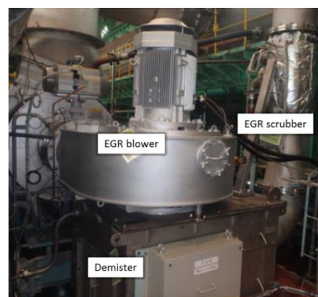
Figure 24. Close up of EGR components
