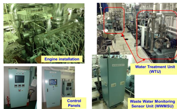
Figure 10. Overview of the installed LP-EGR
